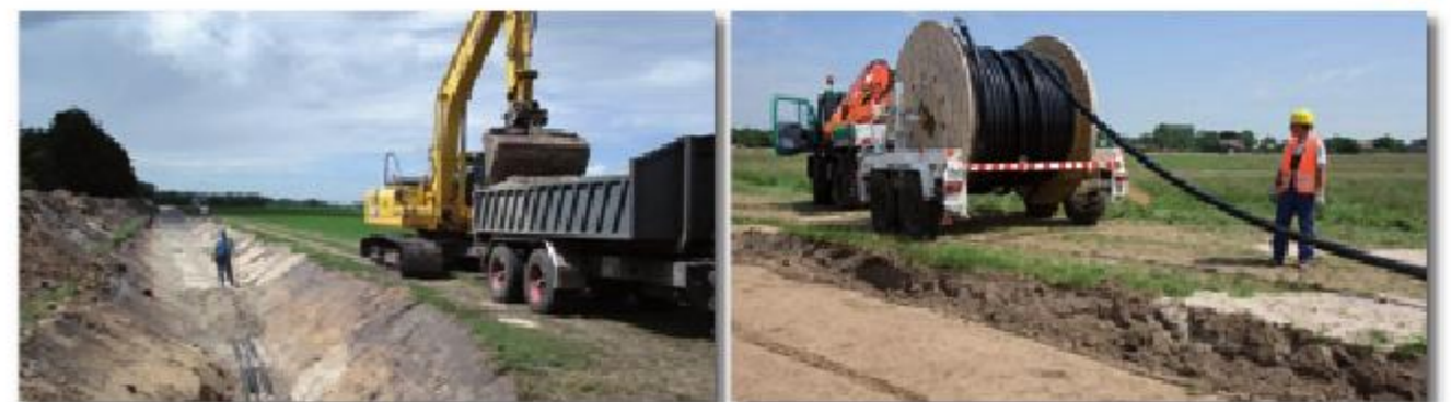
Along with the withstand test, the quality of the cable laying and installation is being increasingly combined with a PD diagnosis (pictures ABB)
